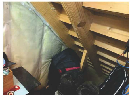
Under Stair At Basement
