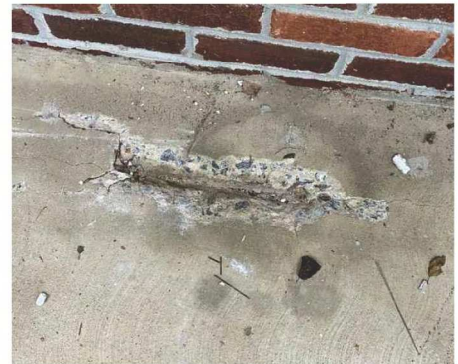
Front Porch Floor
