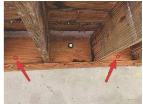
Underside of Deck Left Side Elevation
