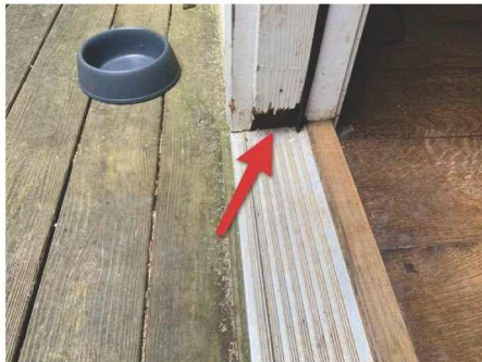
Exterior Door At Dining Room
