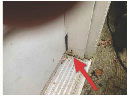
Exterior Door At Dining Room
