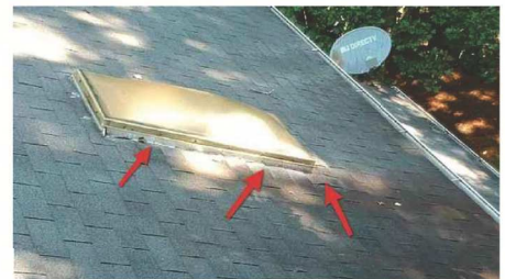
Shingles At Skylight
