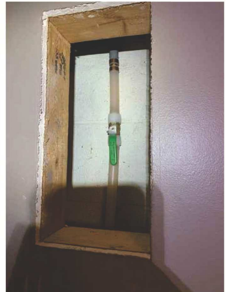
Basement Bedroom Front Wall
