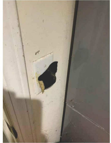
Garage Utility Room
